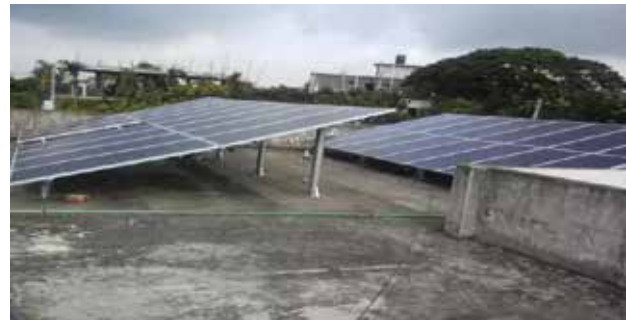
Figure 2: 10 kWp rooftop solar plant with Net metering at Narayanganj PBS-2
